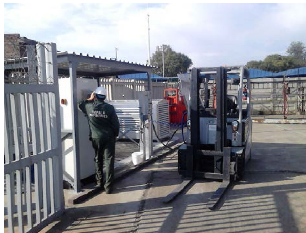
Fig. 21 Simplified layout (left) and general view (right) of hydrogen refuelling station with MH compressor developed by SAIAMC/UWC for Impala Platinum Ltd. (South Africa)
